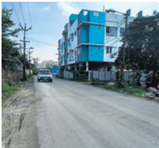
From now on it will be a smooth ride for the two wheelers heading towards Aishwarya Nagar In Ayanambakkam. Though the inner roads were laid sometime back, it was a roller coaster ride leading towards it. It's now a great relief for those residing in that area.
